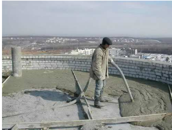
Figure 1. Pouring foam concrete to roofs and walls.
