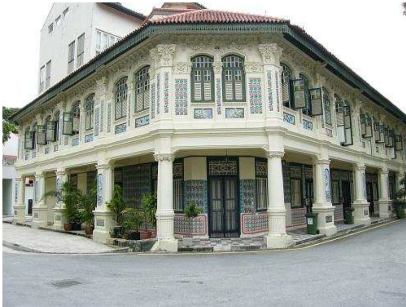
Figure 5. Facade of shop house of Art Deco style.
