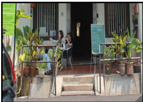
Figure 9: Example from Red Inn Heritage: terracotta tiles with granite steps and a bridge across the drain
