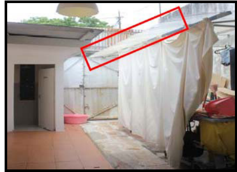
Figure 12: Corrugated polycarbonate as a roof cover for Red Inn Heritage being used as a cover for a clothes drying area
