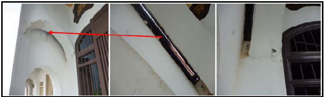
Figure 7: Gap between the left side of Rainbow Lodge and the adjacent building
