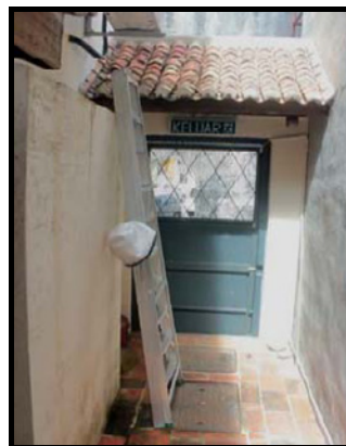
Figure 13: External staircase used as a means of escape to the back lane
