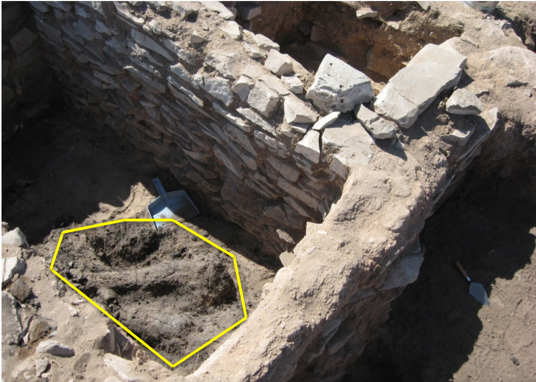
Figure 2.4 Burned Roofing Material at LA 9032 (Frank's Ruin)
