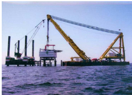
Figure 15: Substation of Horns Rev being installed with an “Asian Hercules” crane. 93
