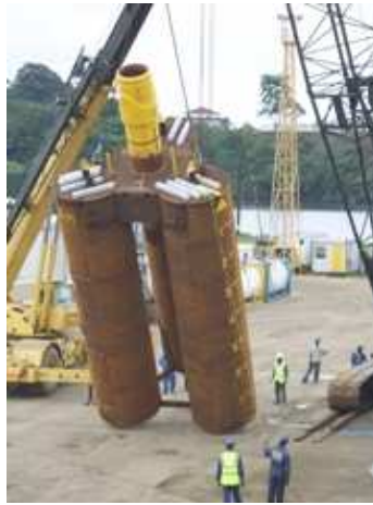
Figure 3: Suction pile cluster. 30
