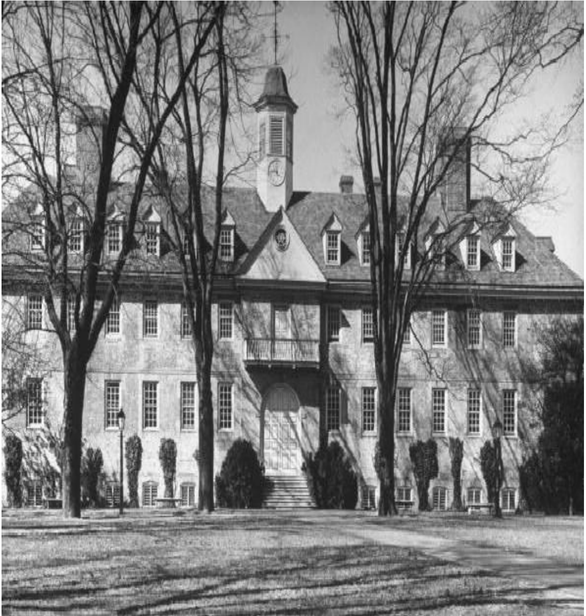
Fig. 2. The Sir Christopher Wren Building, The College of William & Mary (Photograph by Alfred Eisenstaedt, Time & Life Pictures/Getty Images, 31 December 1942)
