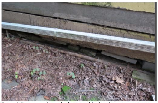
Figure 4. Rotting wood reveals elements of the foundation
