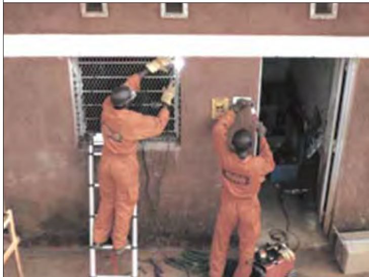
A physical security team improves the security of a police armory's window in BURUNDI.
