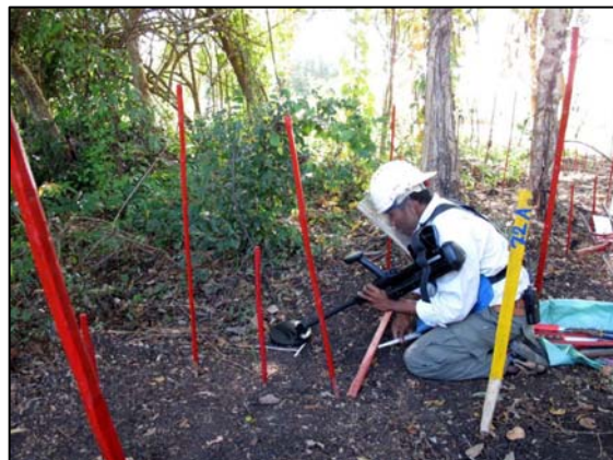
A deminer confirms location of each mine and begins excavation
