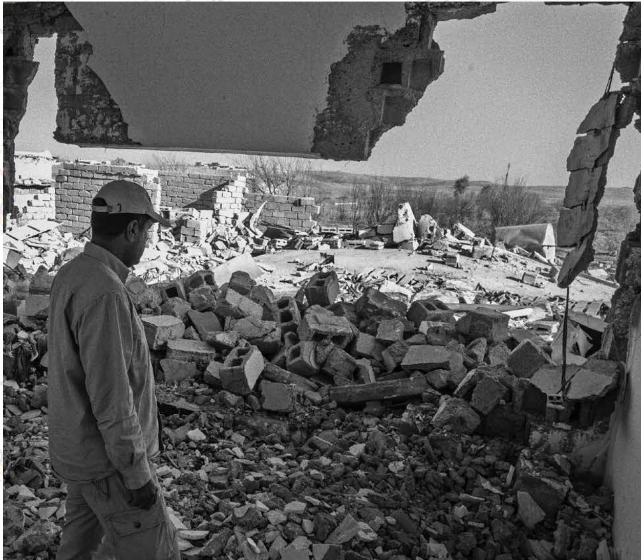
After checking for booby traps in parts of the house still standing, a MAG technical field manager surveys the destruction caused when two villagers set off a booby trap when they opened a door. They were both killed.
