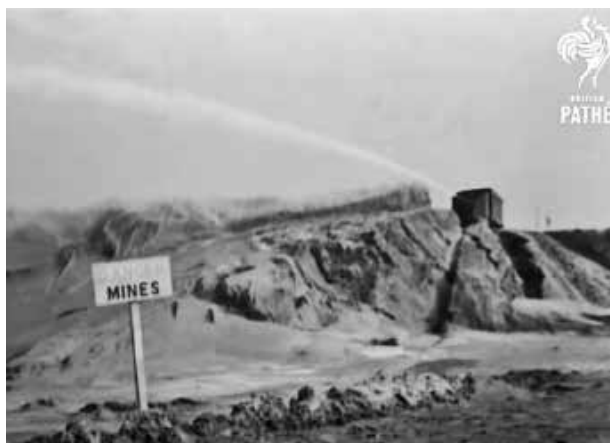
Figure 9. Royal Engineers make use of water jets while clearing Sauntou Sands in Devon, 1947. 21 Figure courtesy of British Pathe.
