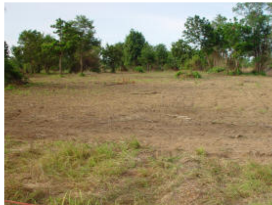
A mechanically prepared area in Thailand. Vegetation is cut and collected, hard soil loosened and the majority of metal contamination removed with the use of a powerful magnet. c/o L. Kaminski
