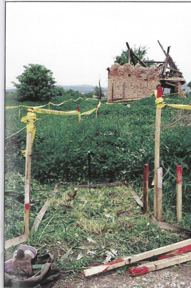
The work station of a deminer: inch by inch safe lanes are cut.
