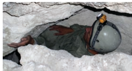
A speleologist inspects an exploded area in order to determine rock condition and its displacement.
