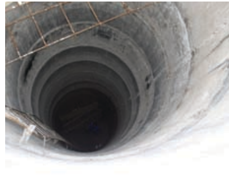
During Stage One, shaft-sinking and tunneling provide underground access. After this step has been completed, stepladders are replaced by special loading equipment.
