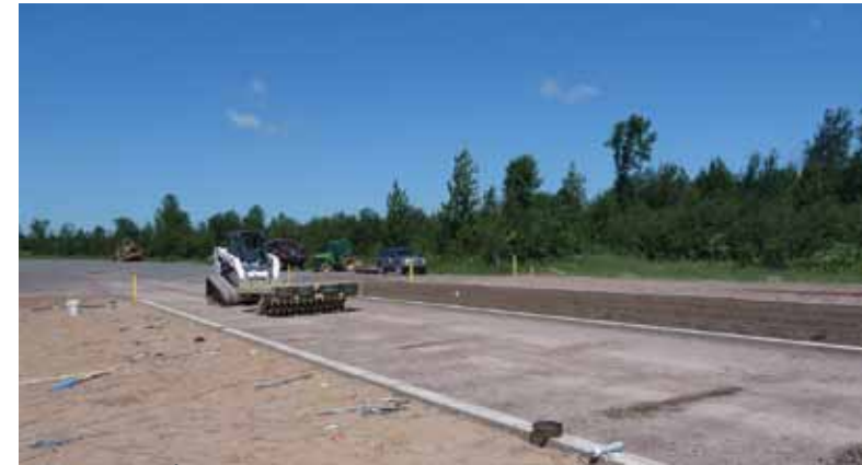
Image 2. SCAMP Roller with Bobcat T-250 prime mover.
