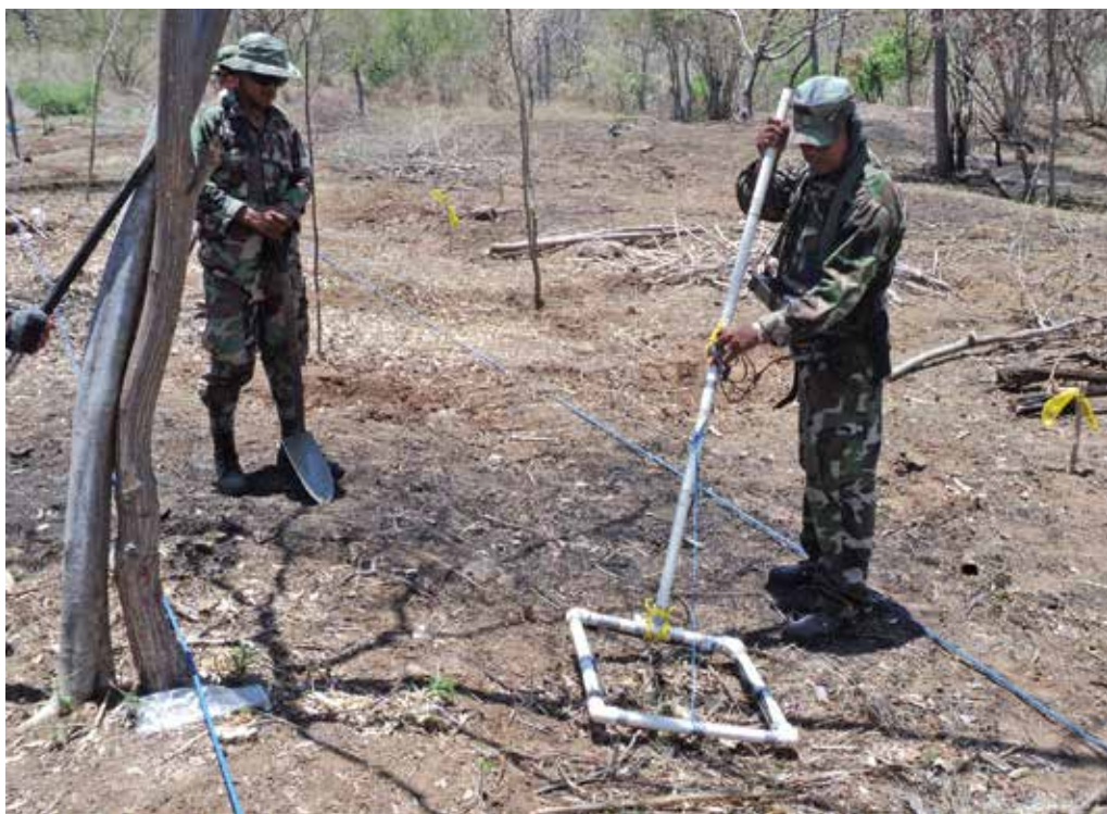
Members of Nicaragua's Army Engineer Corps use UPEX-740 metal detectors to find unexploded ordnance in Chiltepe, Gocen district, Nicaragua.
