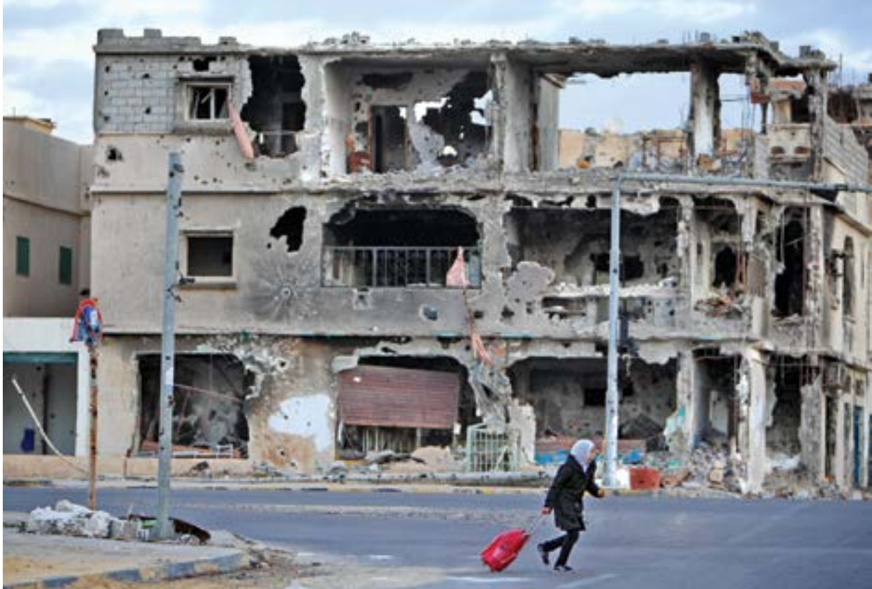
Development takes time in places severely damaged by war such as in Sirte, Libya (2012). Photo courtesy of Giovanni Diffidenti.
