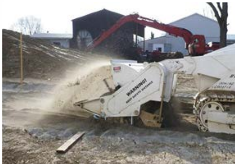
Figure 8. Increased soil turbulence with magnetic roller in lowest position.
