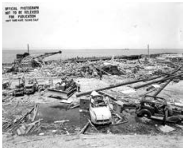
This view looks north, showing the wreckage of building A-7 (joiner shop) in the center and ship pier beyond. A bulldozer and damaged automobiles are seen in the foreground, railway crane at left, and scattered pilings.
