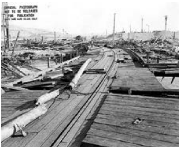
This view looks south from the Ship Pier, showing the wreckage of building A-7 (joiner shop) in the right of the photo. There is a piece of twisted steel plating just to the left of the long pole, left center.
