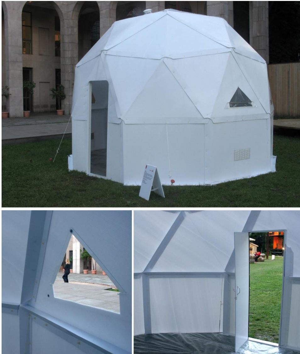
Figure 5. The U-Dome temporary housing system by World Shelters in front the Palazzo dell'Arte of the Milan Triennale.
