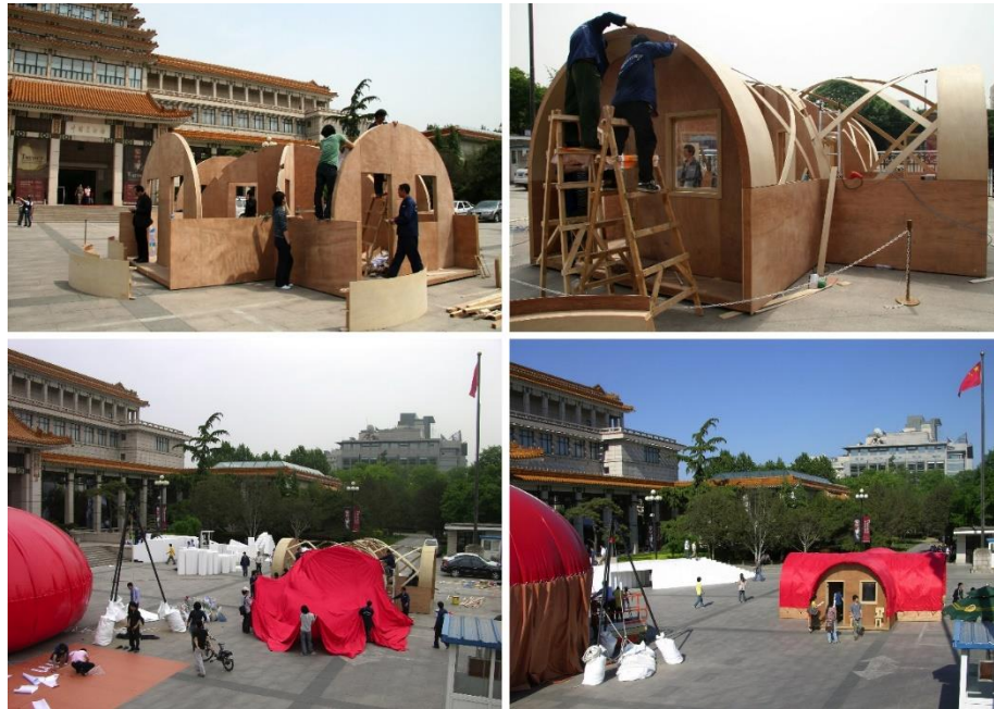
Figure 5. RED+HOUSING, OBRA Architects. Construction phases of the prototype of the project.
