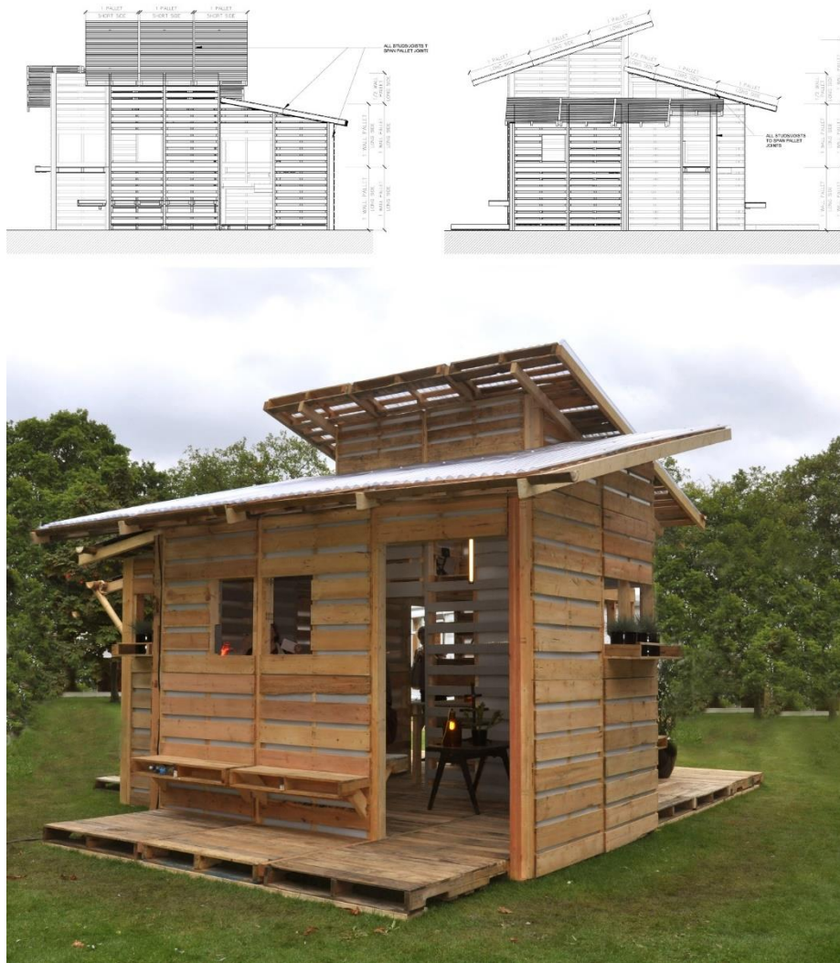
Figure 6. Pallet House, I-Beam Design. Elevations and exterior view of the prototype built in Parco Sempione in Milan.
