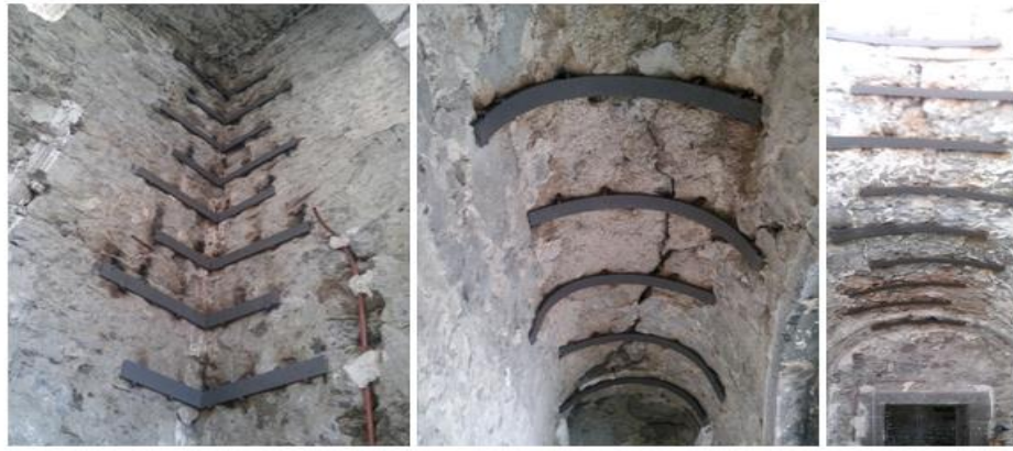
Fig. 5. Strengthening applications
