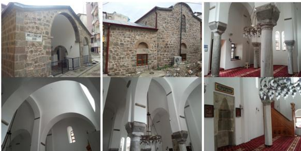
Fig. 9. The images of Molla Siyah Mosque after the restoration
