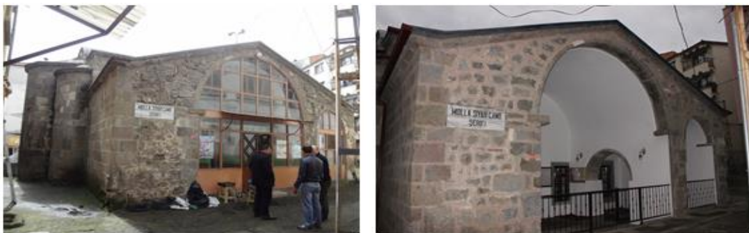
Fig. 2. Images of Trabzon Molla Siyah Mosque before and after the restoration
