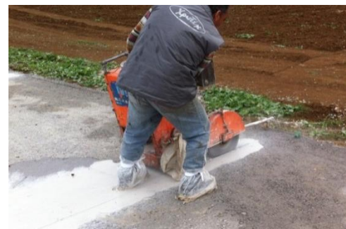
Figure 5 Joint cutting
