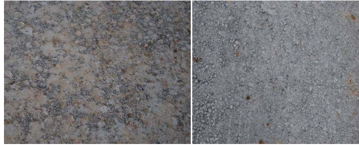
Figure 3 Concrete with limestone on the left and EAF on the right
