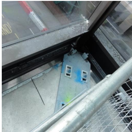
Figure 6 Unitized curtain wall corner bracket
