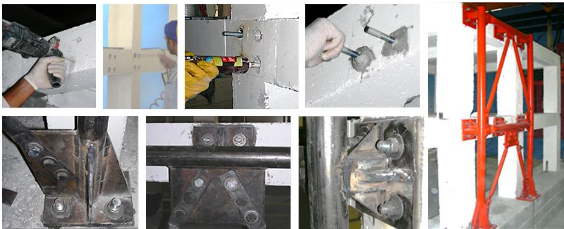
Figure 11 Installation of the External SSW to the RC structure.
