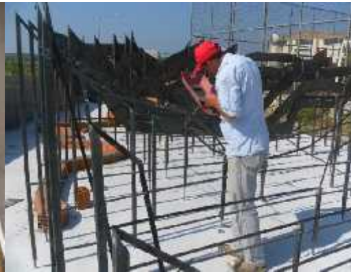
Figure 3b Placing of the sections
