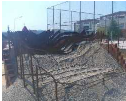
Figure 4 Formation of the concrete surfaces
