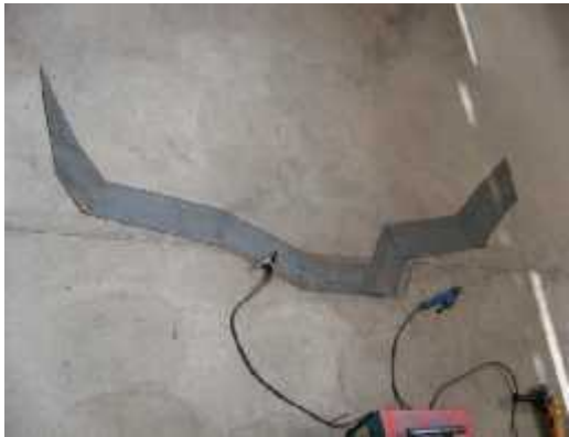
Figure 3a Manufacturing of the sections
