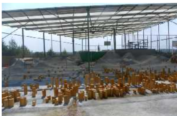
Figure 8a A general view from the downstream part
