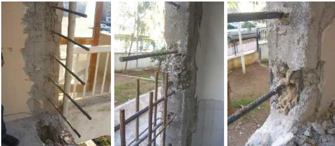
Figure 5 a-b-c. Misapplications of Anchors (photo a-b-c: Ahmet Sari in)
