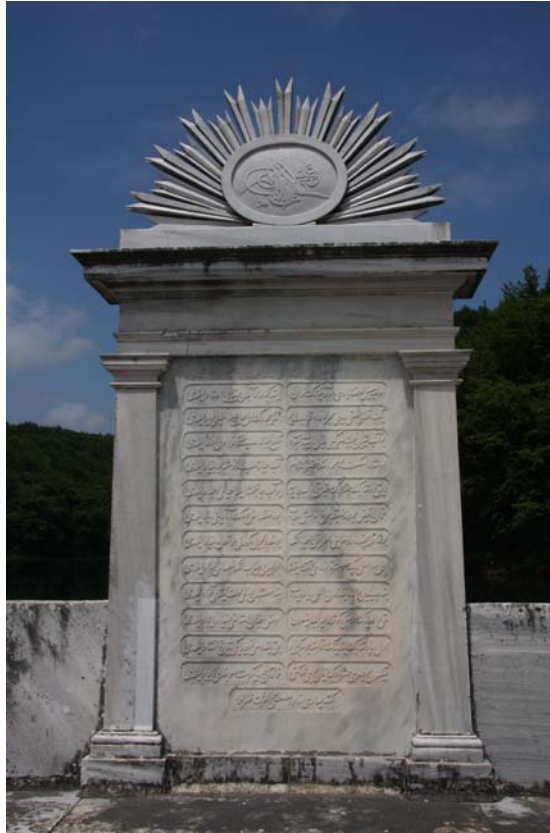
Fig. 2: The Inscription plate of The Sultan Mahmud II Dam
