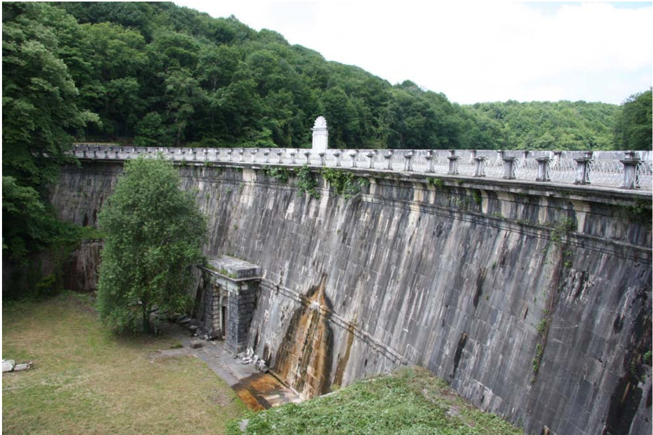
Fig. 3: Downstream Façade of the Sultan Mahmud II Dam
