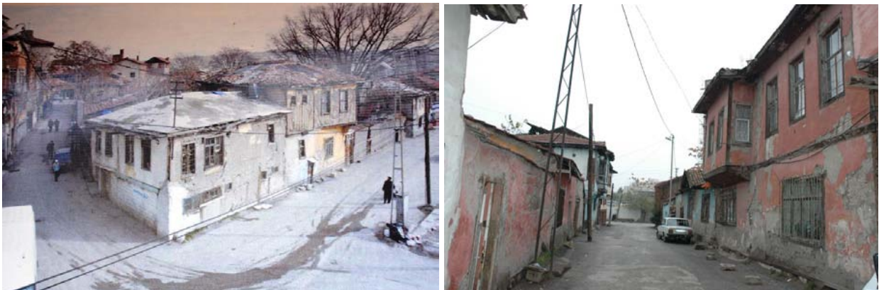
Figure 2, Hamamonu district structure before the rehabilitation project
