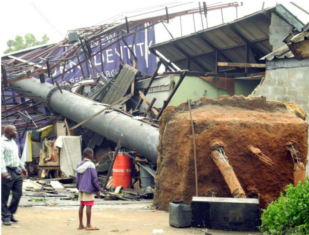
Fig. 4: Rainstorm uproots massive billboard column, Lagos (Source: pnnewsnigeria.com_2011_07_11_aftermath-of-floods-)
