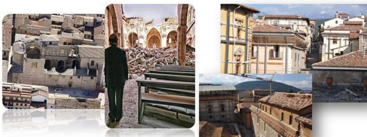
Figure 1: L'Aquila destroyed by the earthquake. On the left, two of the 99 monumental churches of the city. On the right, the whole city under provisory shoring.
