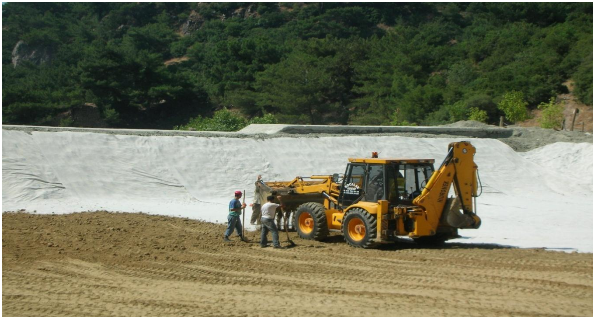
Figure 7. Filling The GCL Layer With A Backhoe
