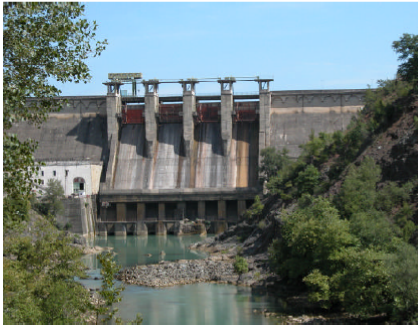
Fig. 1.1 Ulza concrete gravity dam
