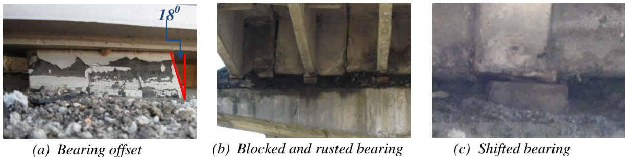
Figure 5 Bearing defects
