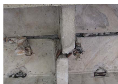
(b) Diaphragm misalignment
