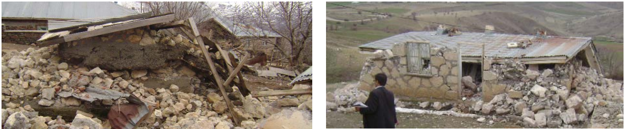
Figure 9 A heavy saddle shape roof
