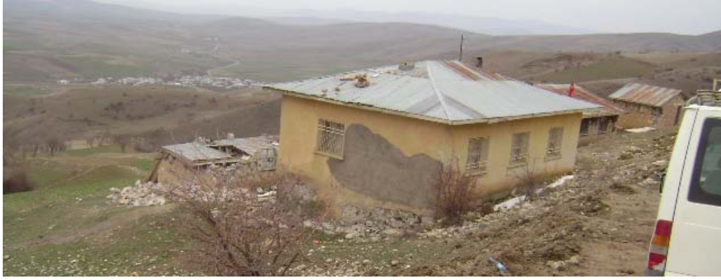
Figure 10 Many of the damaged buildings were located on the hills with a high slope
