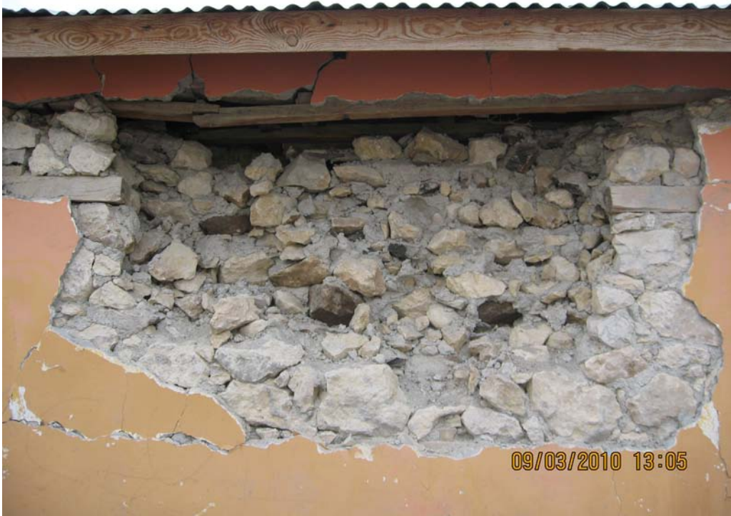
Figure 5 No interlocking element to connect the inner and outer leaves to each other
