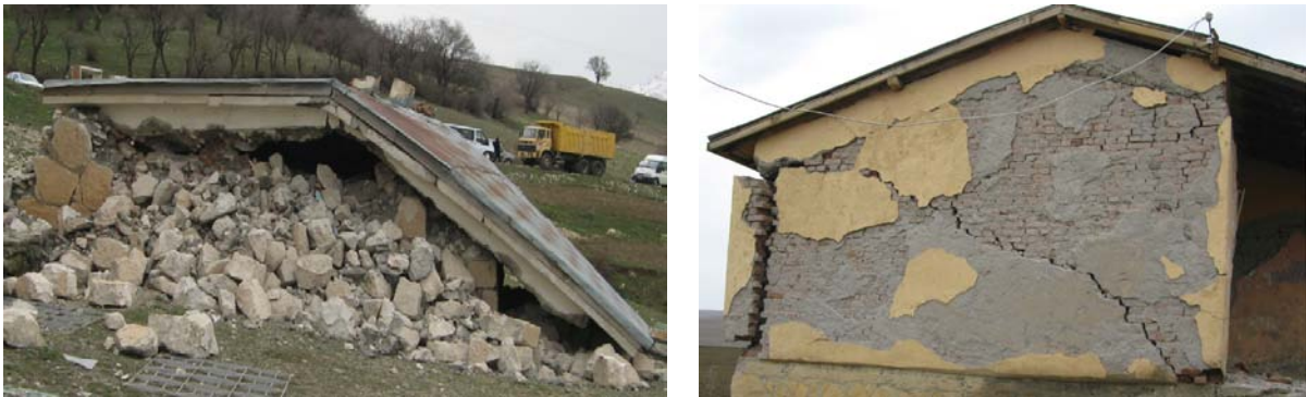
Figure 3 Heavy -saddle shaped roofing systems
