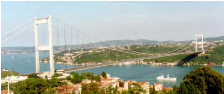
Figure 1 The view of Fatih Sultan Mehmet Suspension Bridge
