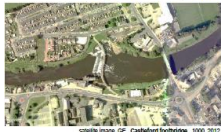
satellite image_of_Castleford footbridge_2002
