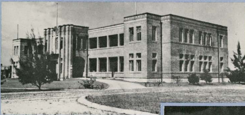
The Administration building at South China Training Institute.
