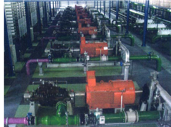
Installation of desalination
