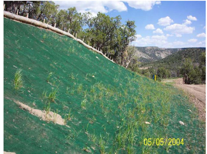
Erosion Control Geotextile for Slope Stabilization
