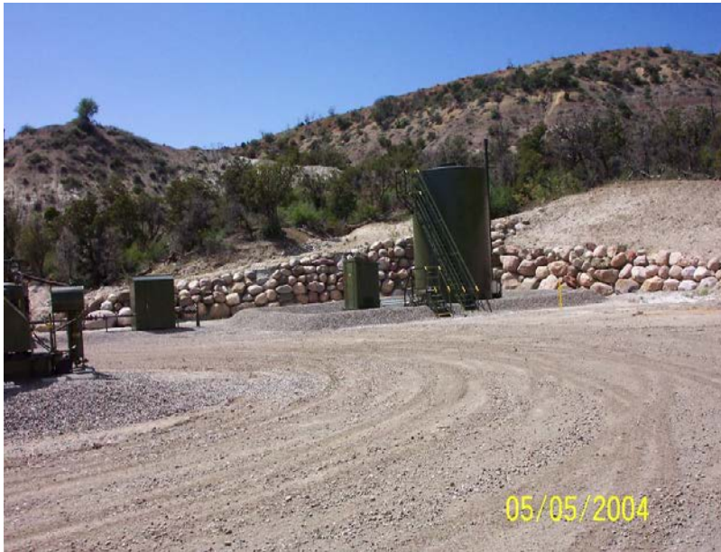
Rock Retaining Wall for Slope Stabilization
