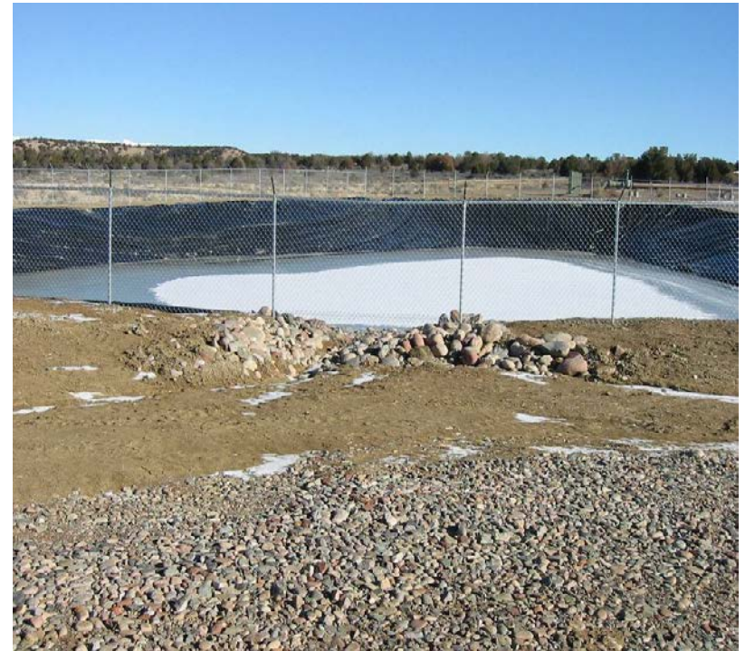
Coyote Gas Plant Storm Water Pond
