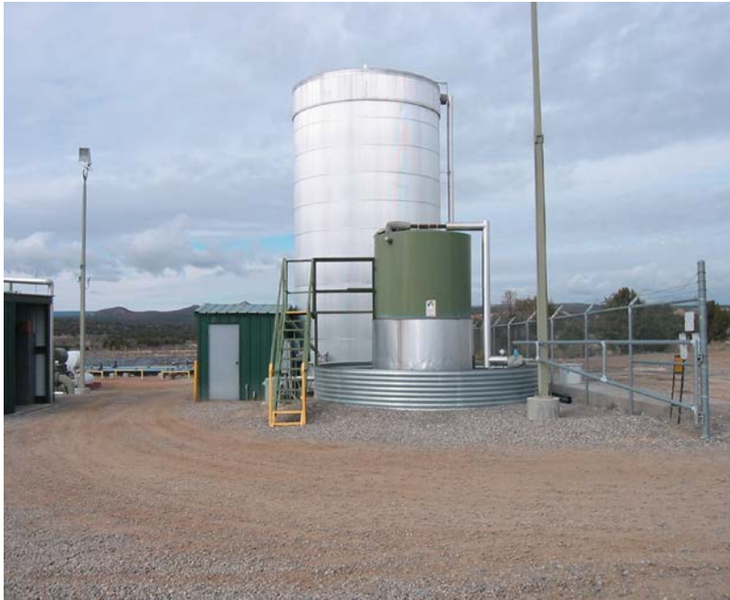
Metal Ring Secondary Containment
