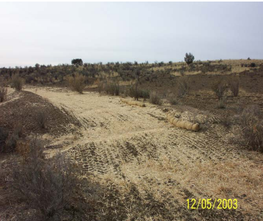
Straw Mulching & Crimping & Erosion Control
