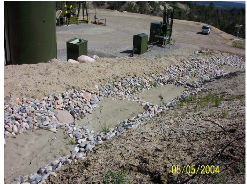
Rock Armored Sediment Control Ditch
