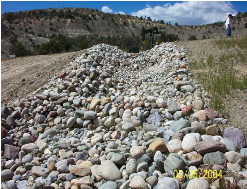
Rock Armored Road Side Ditch
