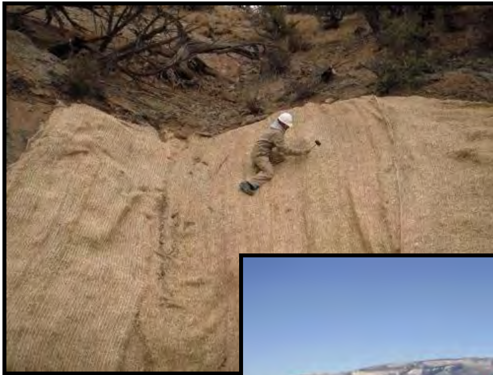
BMP Blanket Install
