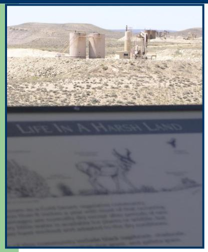
6 coalbed natural gas wells, 2 miles of 2-track road, 2 miles of pipelines and power buried in the road. Can you find it?
