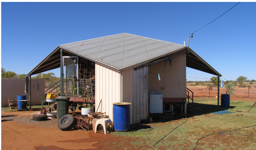
Figure 35: The rainwater collection systems built by a tenant at his Dajarra house provided the main supply of drinking water in 2008. The town bore water was used liberally to maintain a lawn, which reduced dust around the house. (Photo by Tim O'Rourke)
