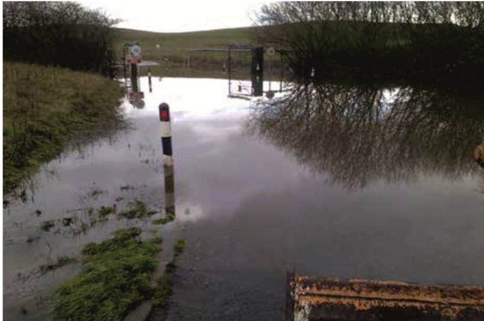
Photograph of September 15 th flooding at Portsea. Source: PCC. Estimated water depth (0.5m – 0.7m).
