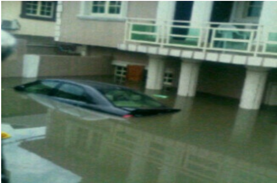
Photograph of July 11 th flooding at Victoria Island. Estimated water depth (1.5m – 1.7m).
