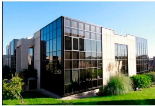
Figure 1. Office reference building under investigation. Latitude: 40.31°N, Longitude: 3.38°W. Location: Madrid, Spain.
