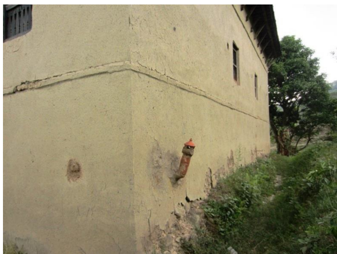
Figure 7: Chimney to ICS in Figure 6
