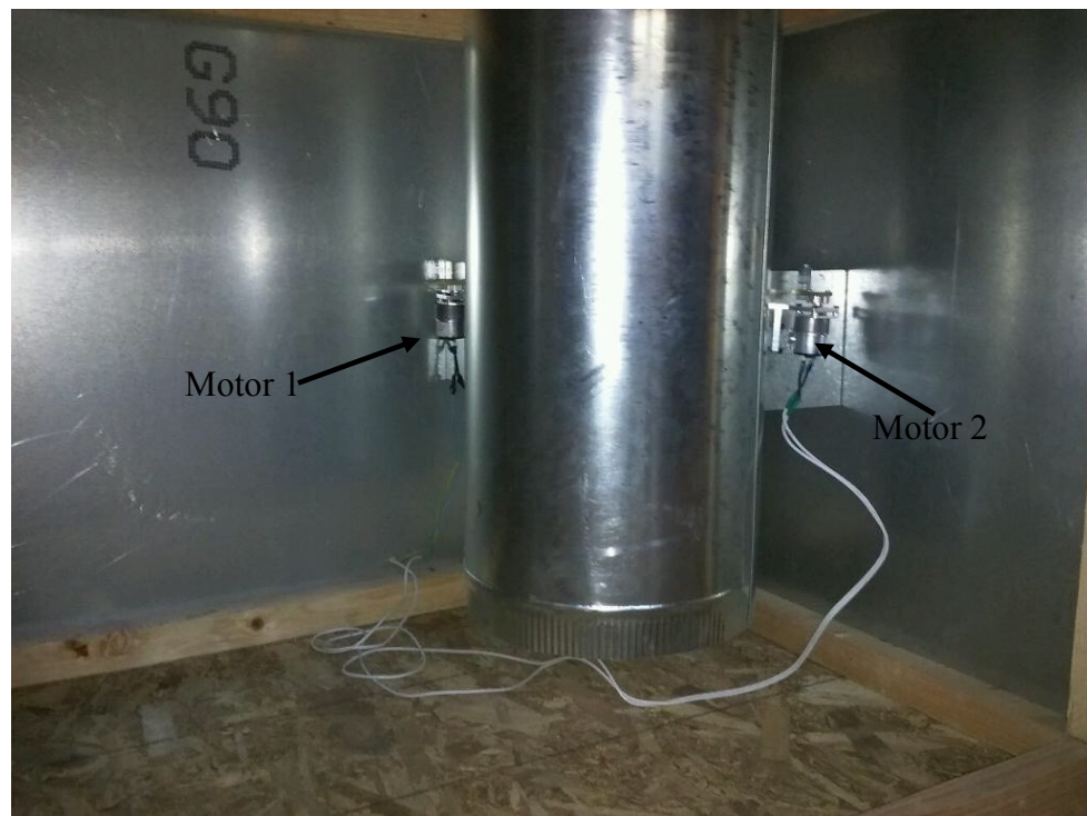
Fig. 7.5. Picture showing two motors firmly attached with the connecting plates and concealed within the doghouse.
