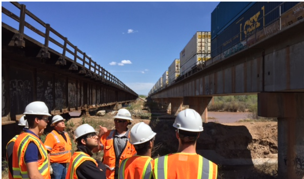
Fig. 1.3. Railroad bridge visual inspection.
