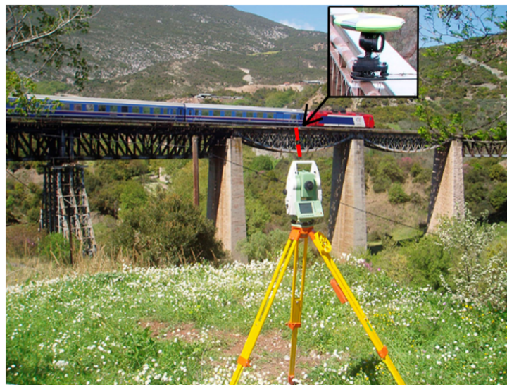
Fig. 2.3. Measurement of the deflection of a railroad bridge using a RTS (Psimoulis and Stiros, 2013).
