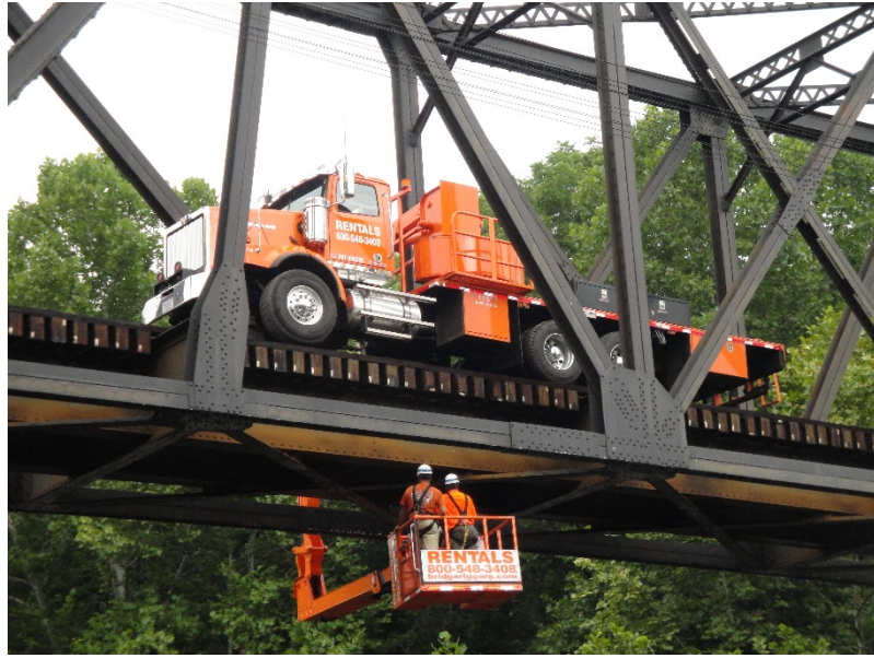
Fig. 2.1. Crane-aided visual inspection of railroad bridge (N.E. Bridge Contractors 2016).
