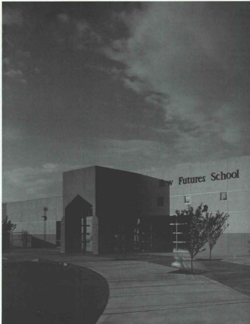
New Futures School, Northeast Facade.
