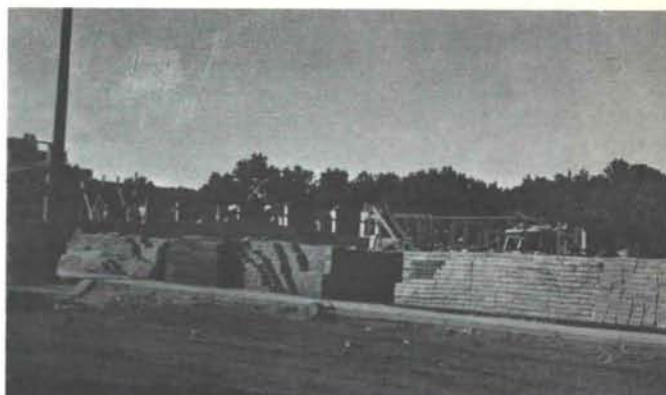
fig. 1 early stage of construction with west wing on the left.
