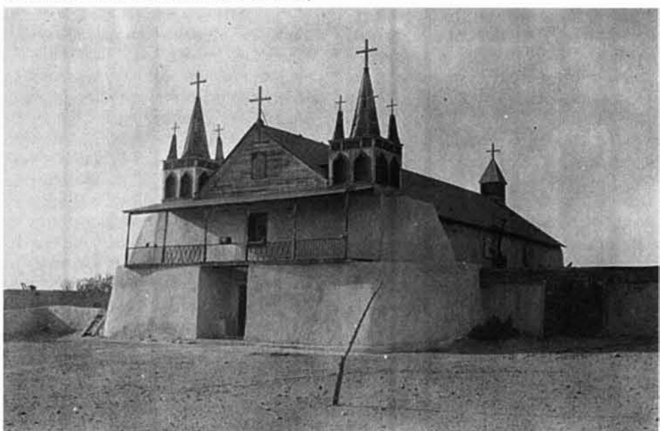
San Agustín de la Isleta Mission, built of terrones, with wooden Gothic Revival elements Photograph taken in 1925.
