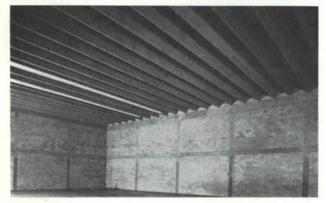
New 10,000 square foot fireproof warehouse facility for All Points Movers, Division of Southwest Moving and Storage Co., featuring the new 8' wide twin tee prestressed concrete members spanning 74' with U. L. two hour label.
